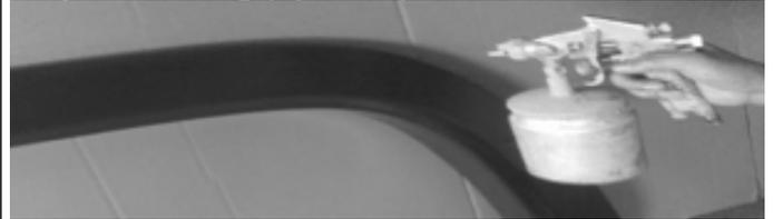
Professional paint or body shop recommended to paint flares. Follow all the paint manufacture specifications to paint the flares. Clean fender flare surfaces with clean water and a mild detergent before painting, do not use lacquer thinner or any solvent based products.
